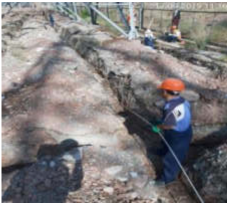
Picture 8. Installation of ground conductor (Status in September 2019)
