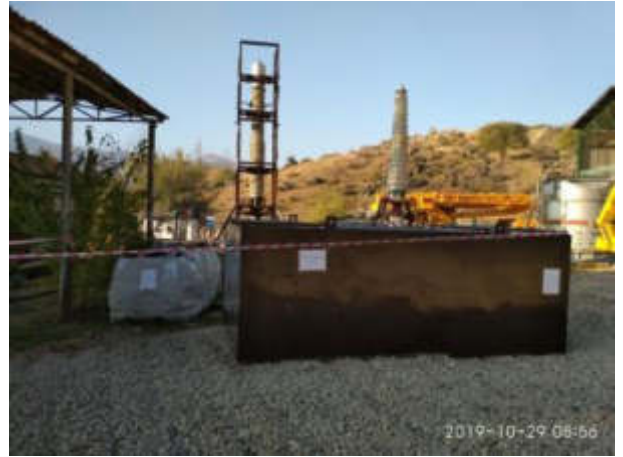
Picture 19. A new container for temporary storage of asbestos containing material (Status in October 2019)
