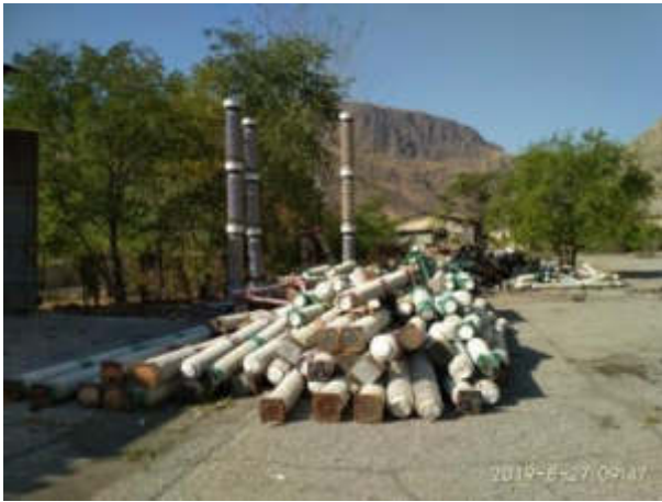
Picture 28. Ceramic waste was stored at storage area of the Cascade of Toktogul HPPs (Status in August 2019)
