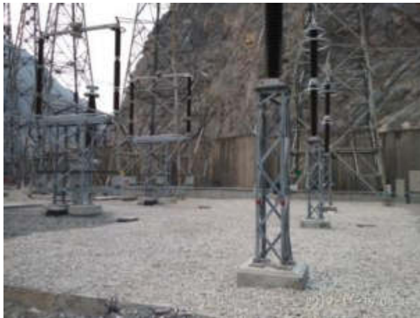
Picture 20. 500 kV transition point after covering with gravel (Status in November 2019)
