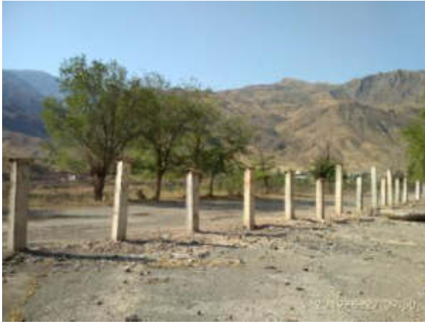
Picture 26. Old concrete poles were reused for fencing at the Cascade of Toktogul HPPs (Status in August 2019)
