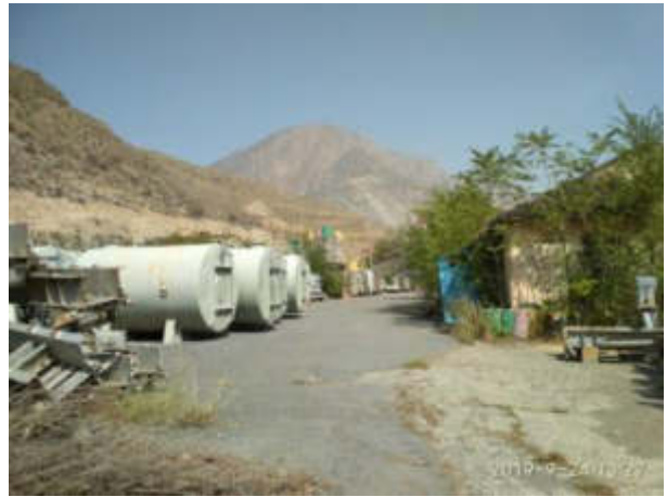
Picture 29. Scrap metal and old dismantled equipment were stored at the fenced storage area of the Cascade of Toktogul HPPs (Status in September 2019)
