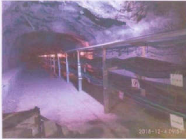
Pic.1. Area of 500 kV Cabel tunnel of Toktogul HPP
