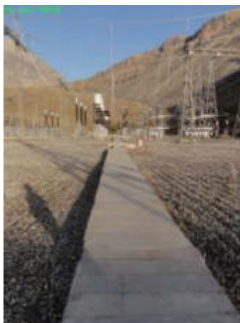
Picture 12. New cable duct within switchyard site (Status in October 2019)
