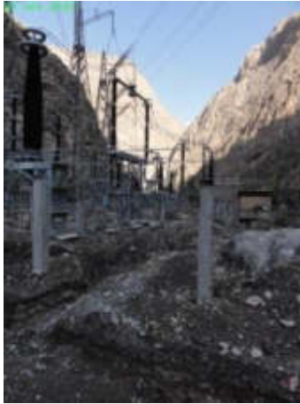
Picture 18. Last electric grounding works at transition point (Status in October 2019)
