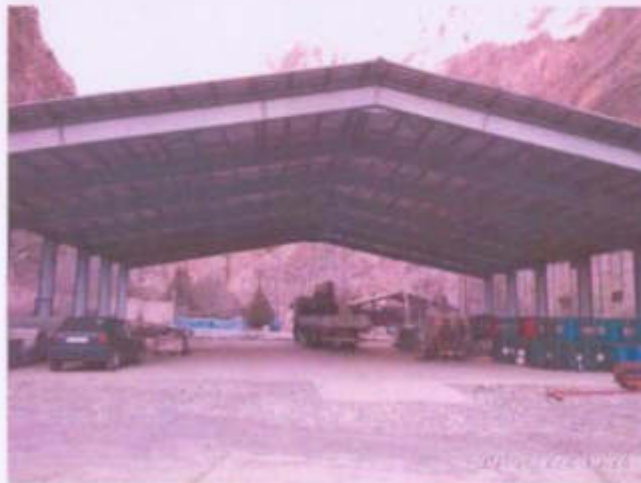
Pic.3. Area of the Oil storage of Toktogul HPP
