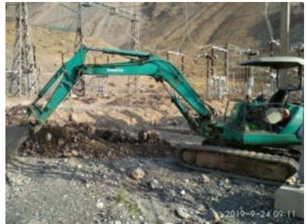
Picture 9. Earth works at 500 kV substation (Status in September 2019)
