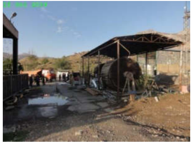
Picture 15. Waste remnants on switchyard site (Status in October 2019)
