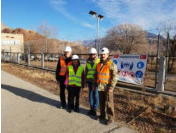
Picture 34. PIC and PIU specialists are inside of the fenced and protected area of 500 kV Substation of Toktogul HPP (Status in March 2019)
