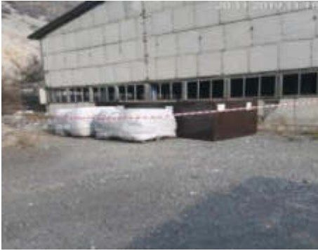
Picture 22. Containers with asbestos waste were transported to storage area of the Cascade of Toktogul HPPs (Status in November 2019)
