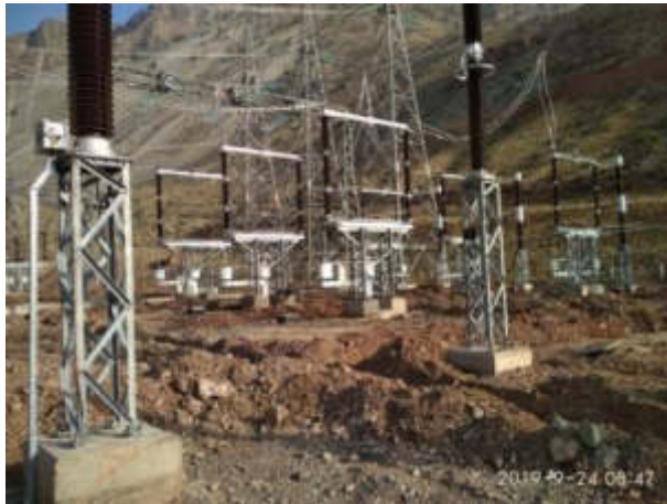
Picture 10. Works on ground conductor (Status in September 2019)
