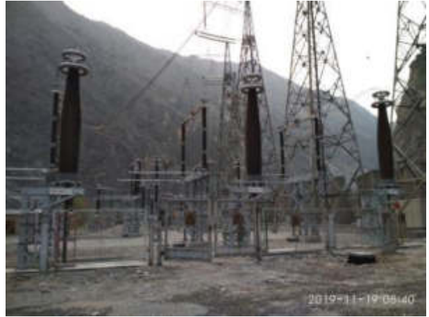
Picture 23. 500 kV Transition point after rehabilitation works (Status in November 2019)
