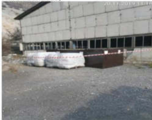
Pic.3. Containers with asbestos containing waste placed at the Client's/Cascade of THPPs storage site (Status in November 2019)
